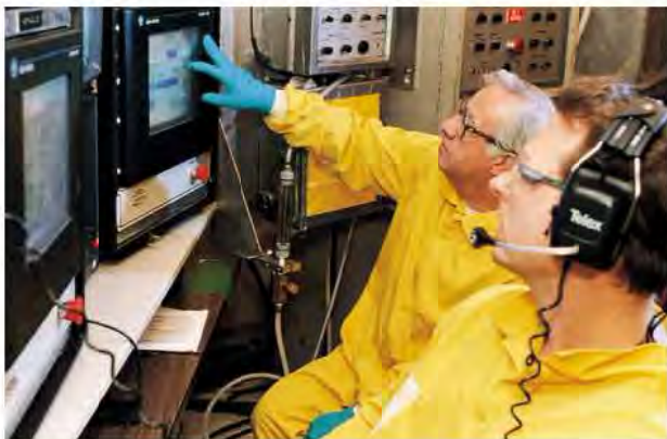
FTI baffle bolt inspection rates have been faster than realized on previous baffle bolt deployments, in part because tooling was re-designed by FTI to be multi-functional, saving setup and delivery times.
